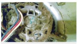
A dirty, inefficient blower caused by air bypass from a 1" filter.
