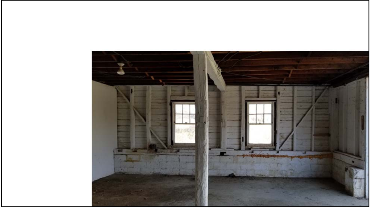
This in the interior view of the garage.
