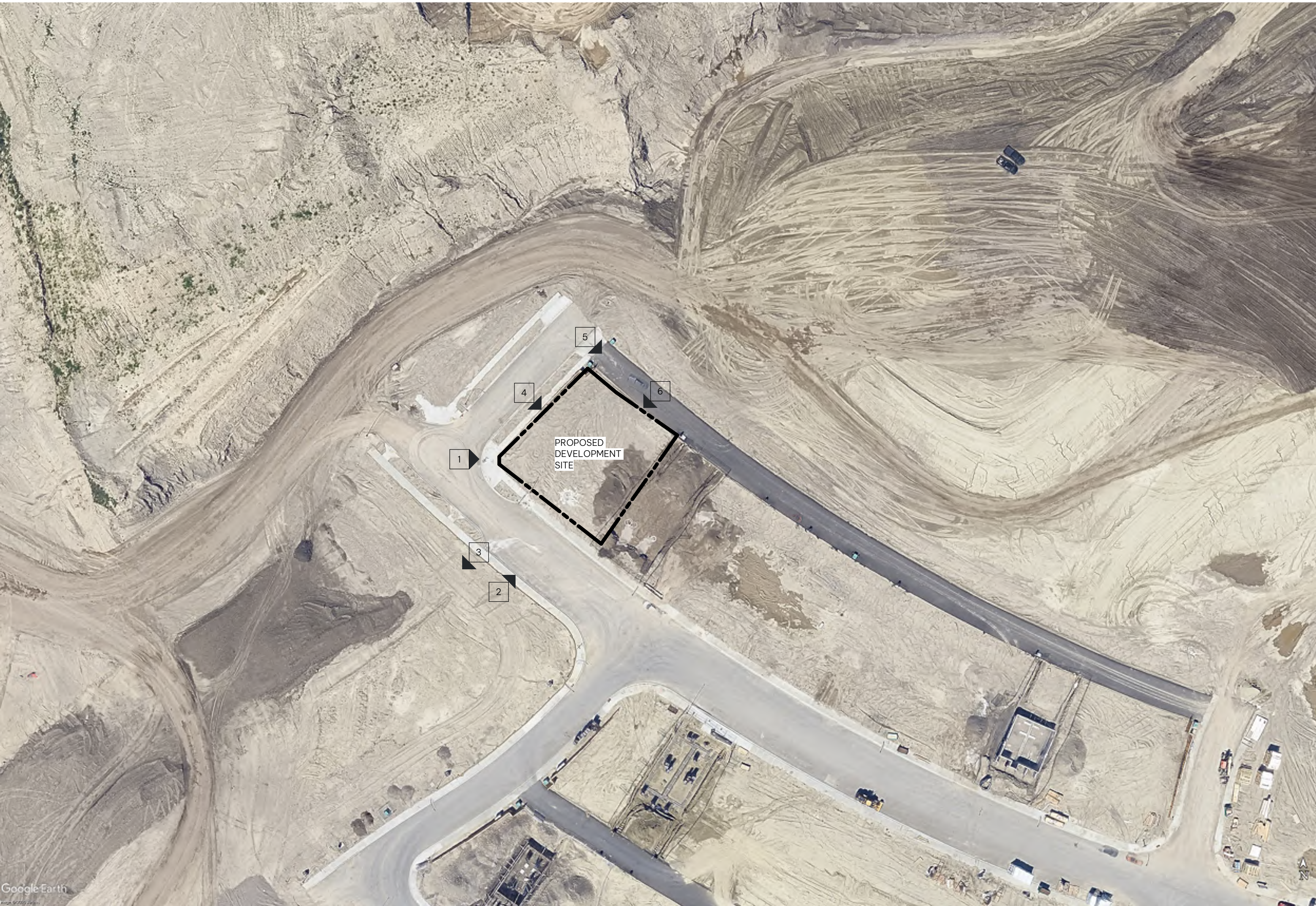
7 Aerial Site View
