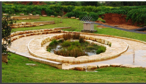
Israel's first stormwater bio-filtration system, was built by KKL-JNF in Kfar Saba. (Courtesy of The Center for Water Sensitive Cities in Israel)
