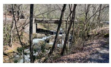
There are dozens of bridges that you have to pass as you go down the bike trail. They are all well maintained. The only alert you need to have is at each end. Erosion will have lowered the bike trail sometimes up to 6 inches from the edge of the bridge. There is either a sudden drop or a bump as you go up on the bridge deck planks. But these low spots are easy to succumb.
