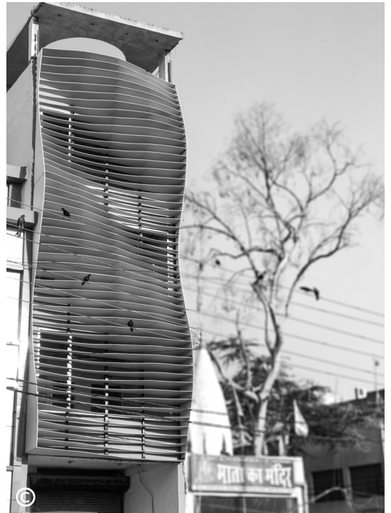
3. Exterior view during construction phase, showing panel distribution in main facade
