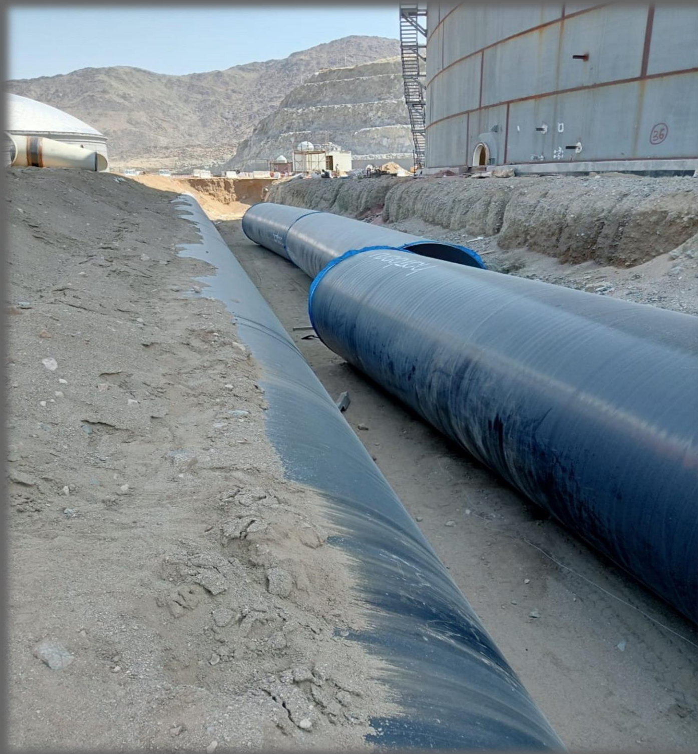
Welding of 88" & 100" CS Pipe
