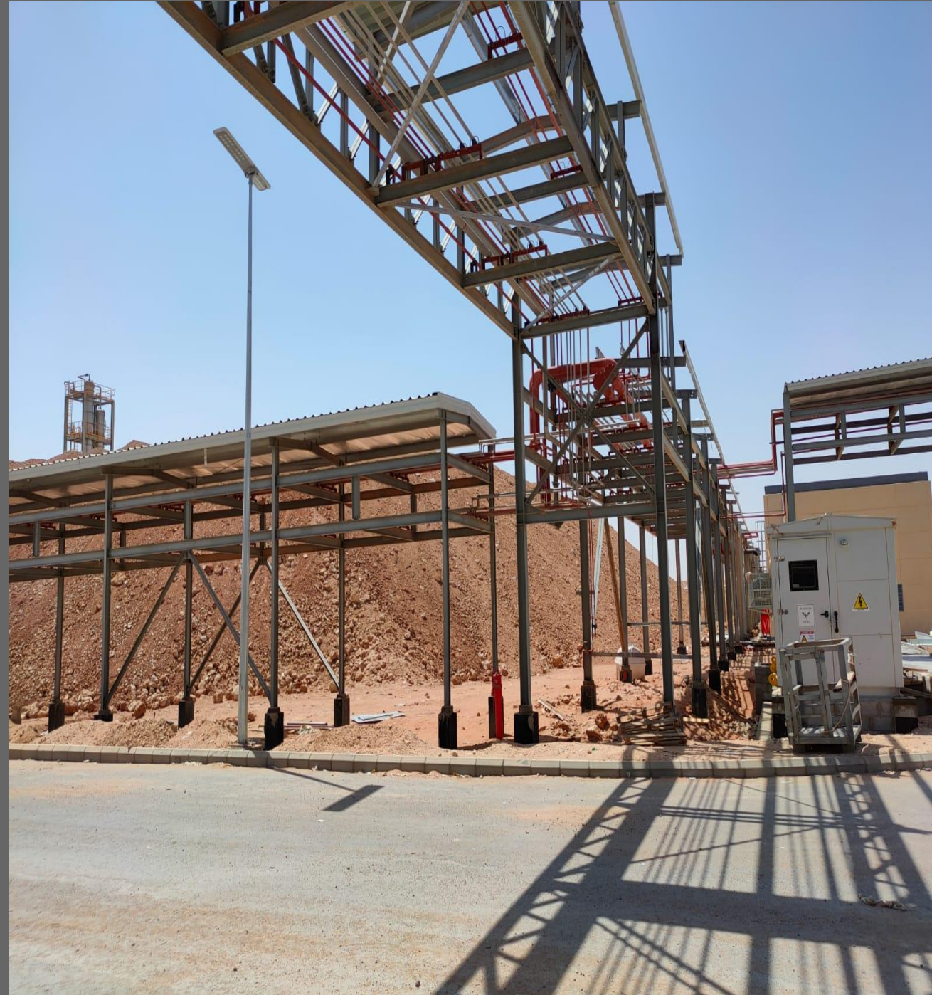
Fire Steel Storage With SS Piping Rack system
