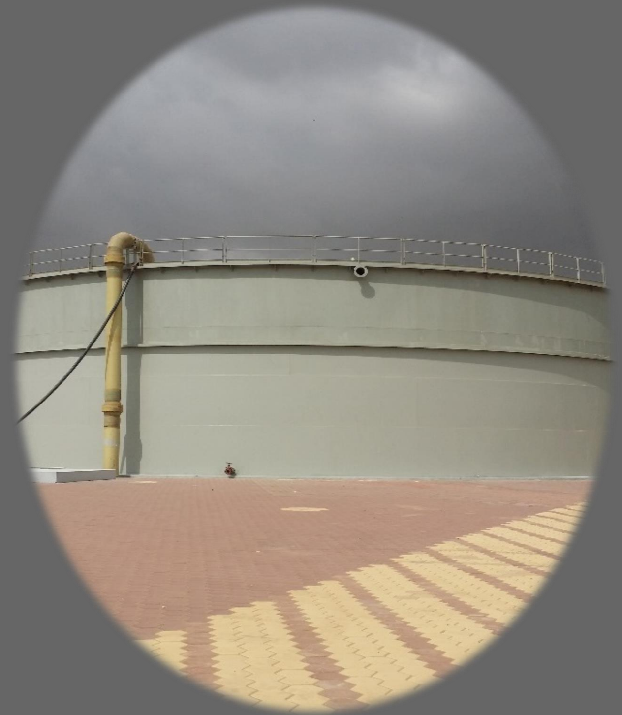
Steel Storage Tank 7,000m 3 Dia: 33.00m
