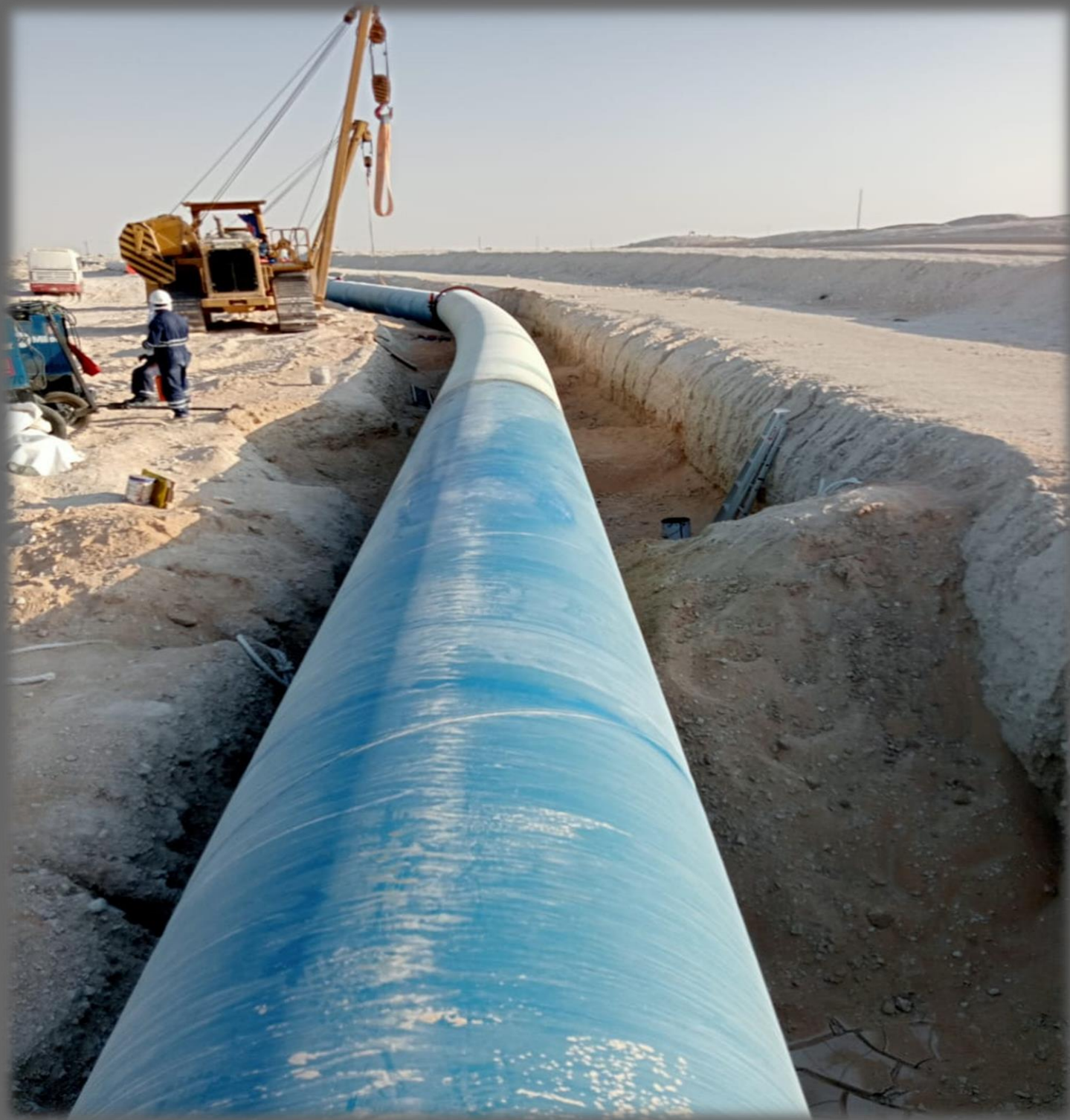
Welding of 56" CS Pipe
