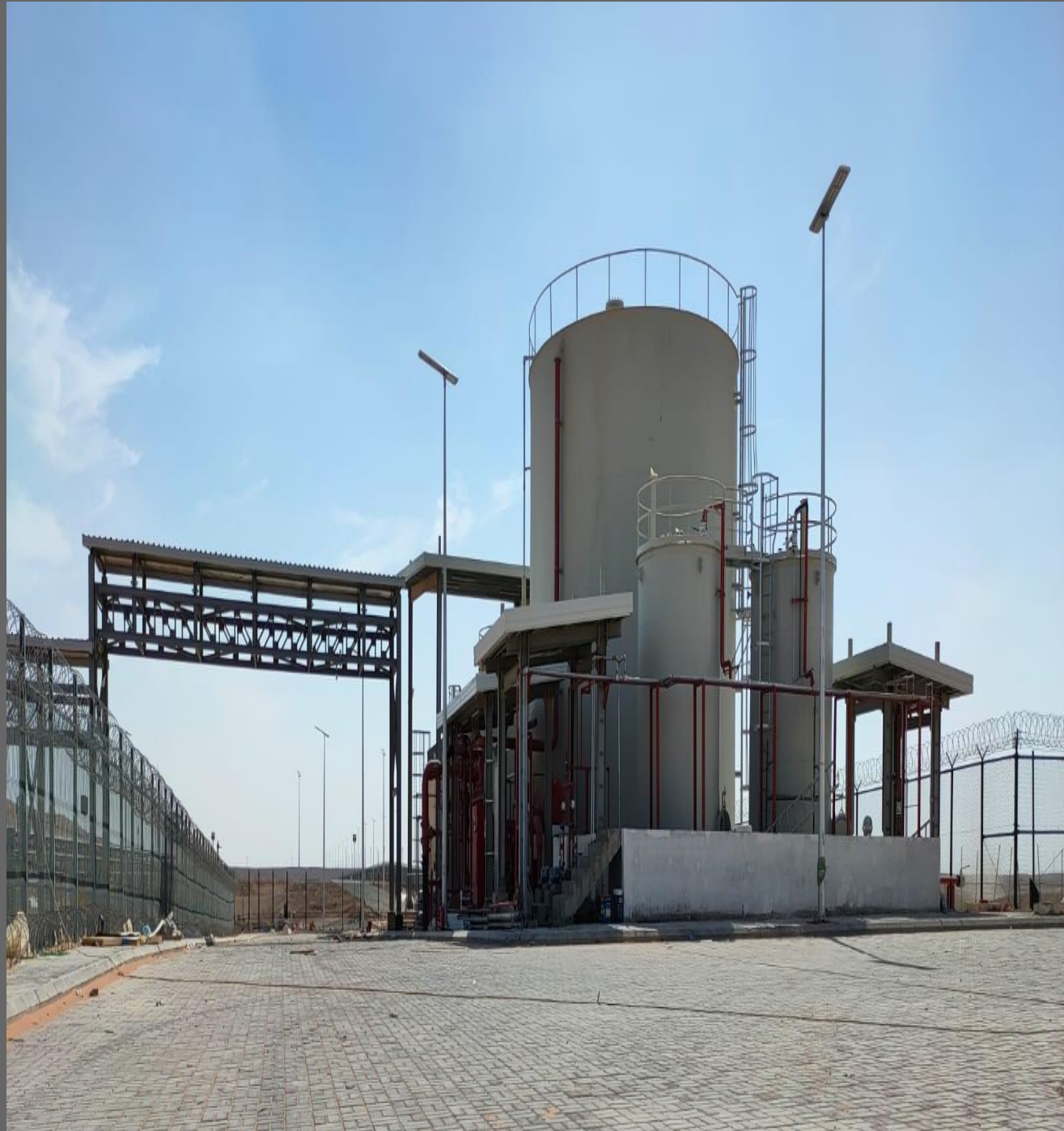
Fire Steel Storage With SS Piping Rack system
