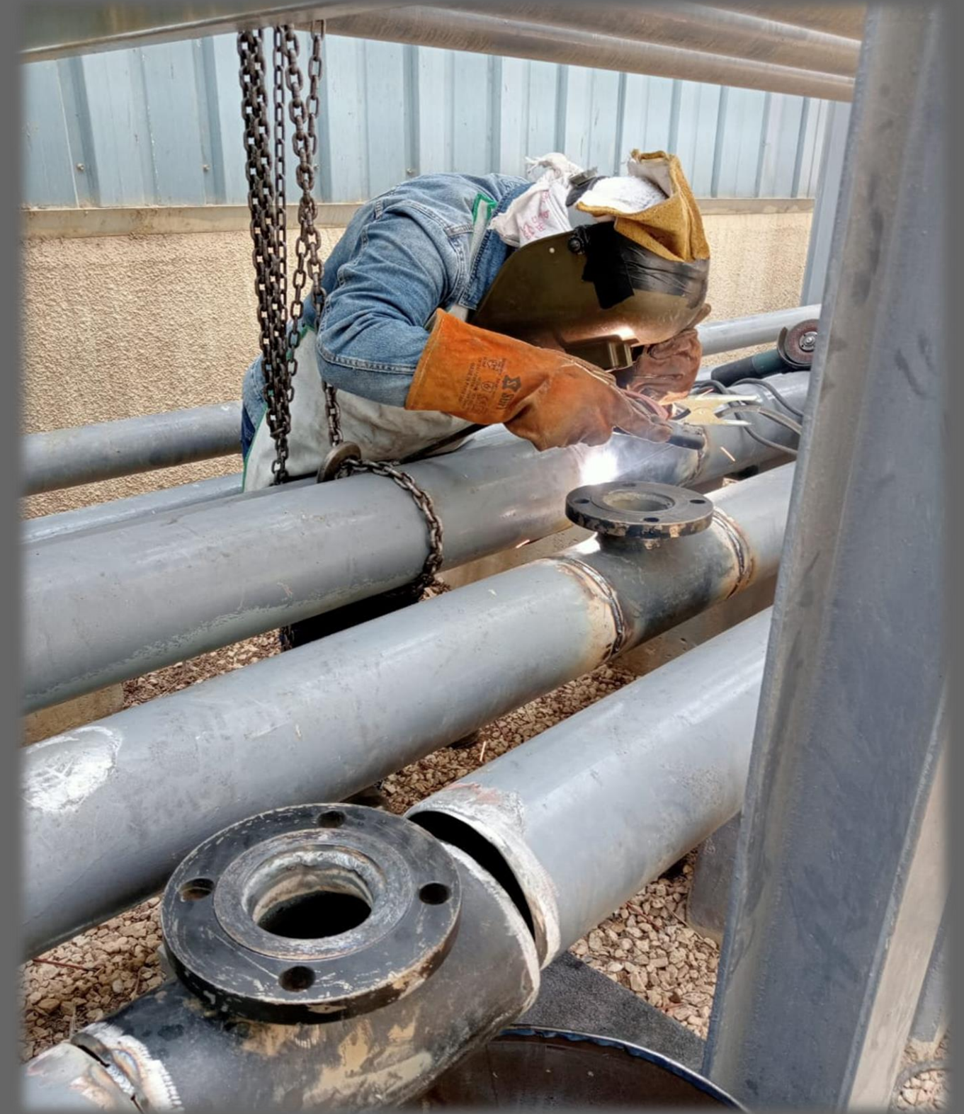
Petromin Shutdown Piping work
