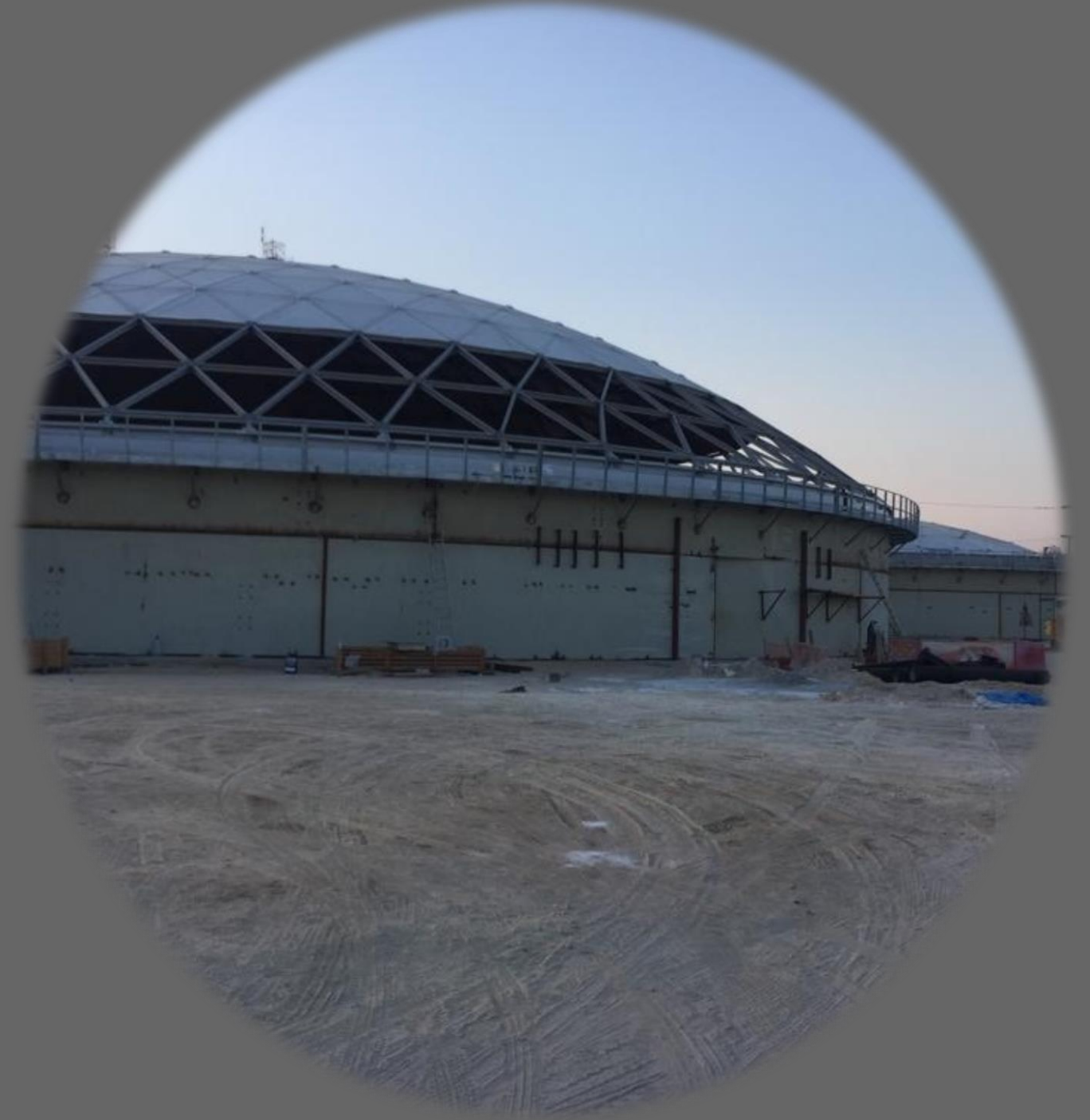
Erection of Steel Storage With AL Dome Roof by Hydraulic jacks. Tank 27,000m 3 , Dia: 56,64m
