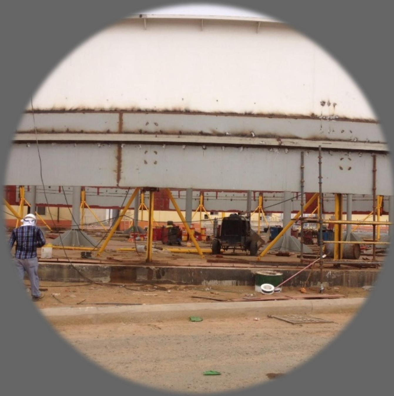
Erection of Steel Storage by Hydraulic jacks. Tank 7,000m 3 , Dia: 33.00m
