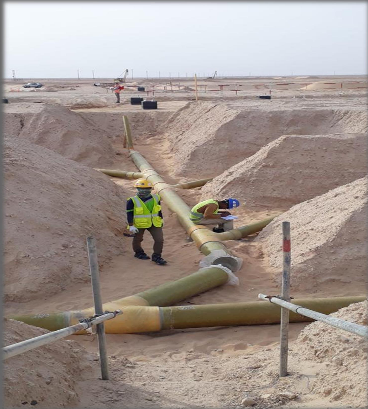
GR Pipe Installation
