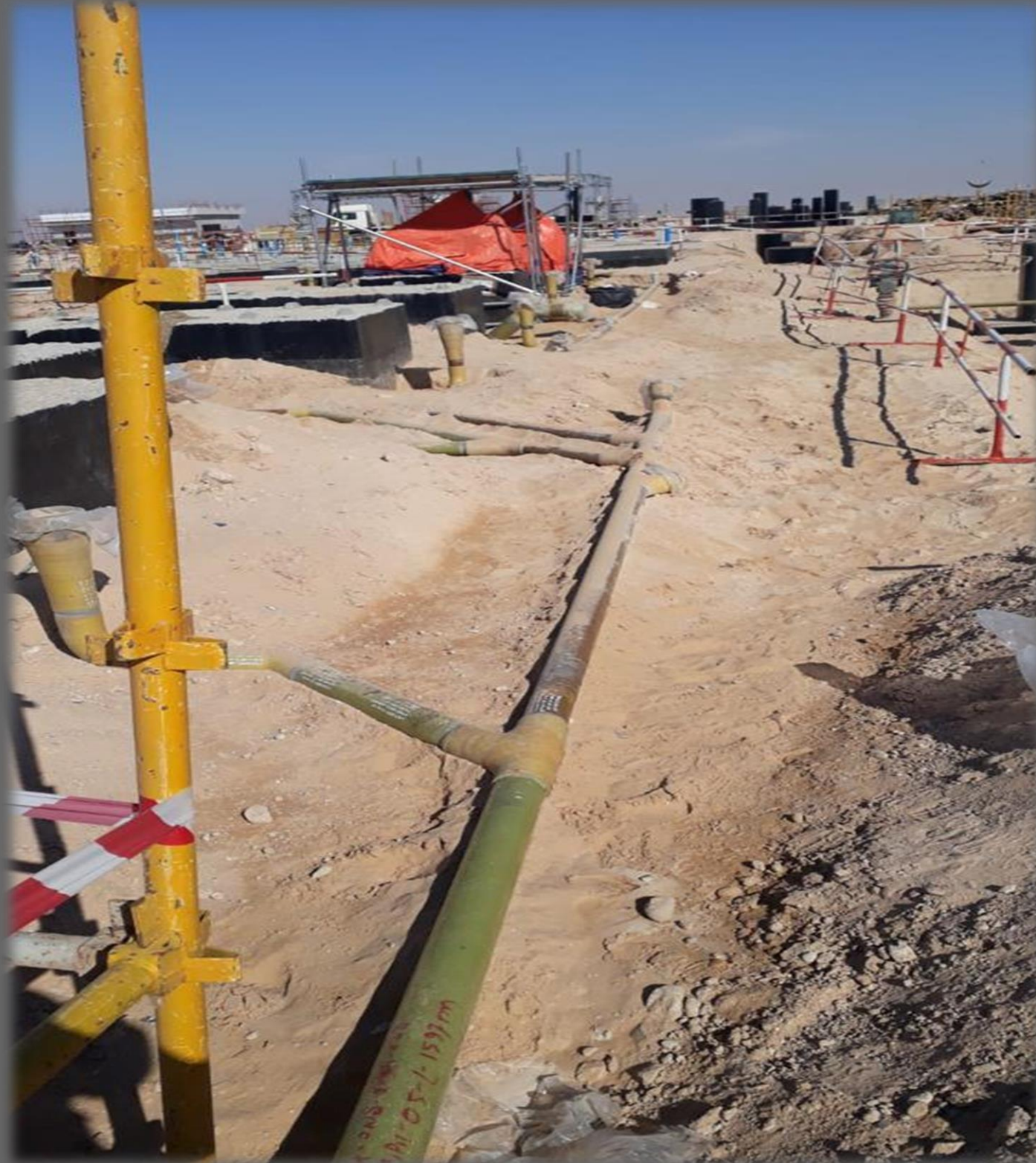
GR Pipe Installation
