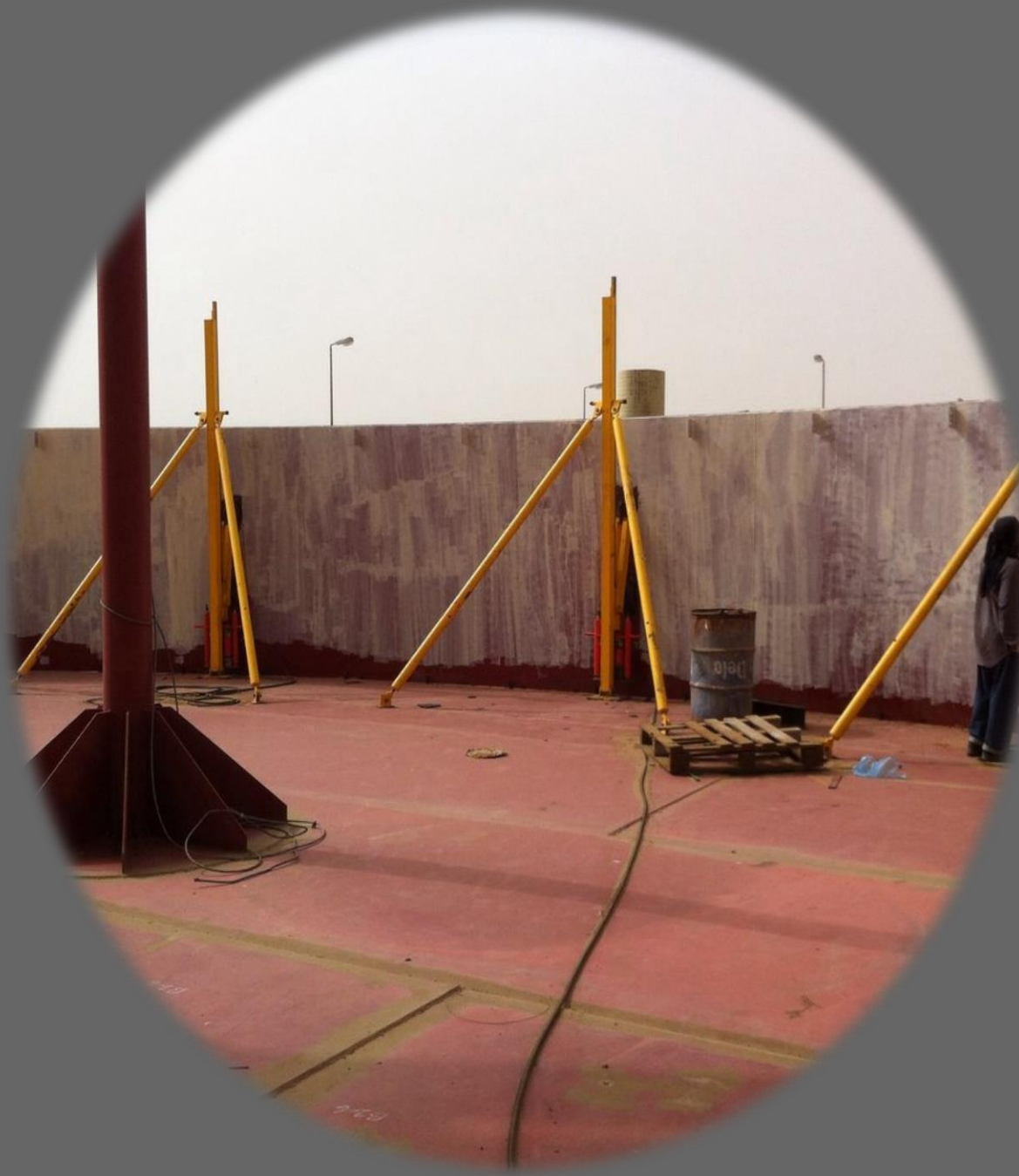
Erection of Steel Storage by Hydraulic jacks. Tank 5,000m 3 , Dia: 27.23m
