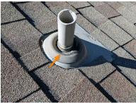
Right - inverted rubber boot flashing
