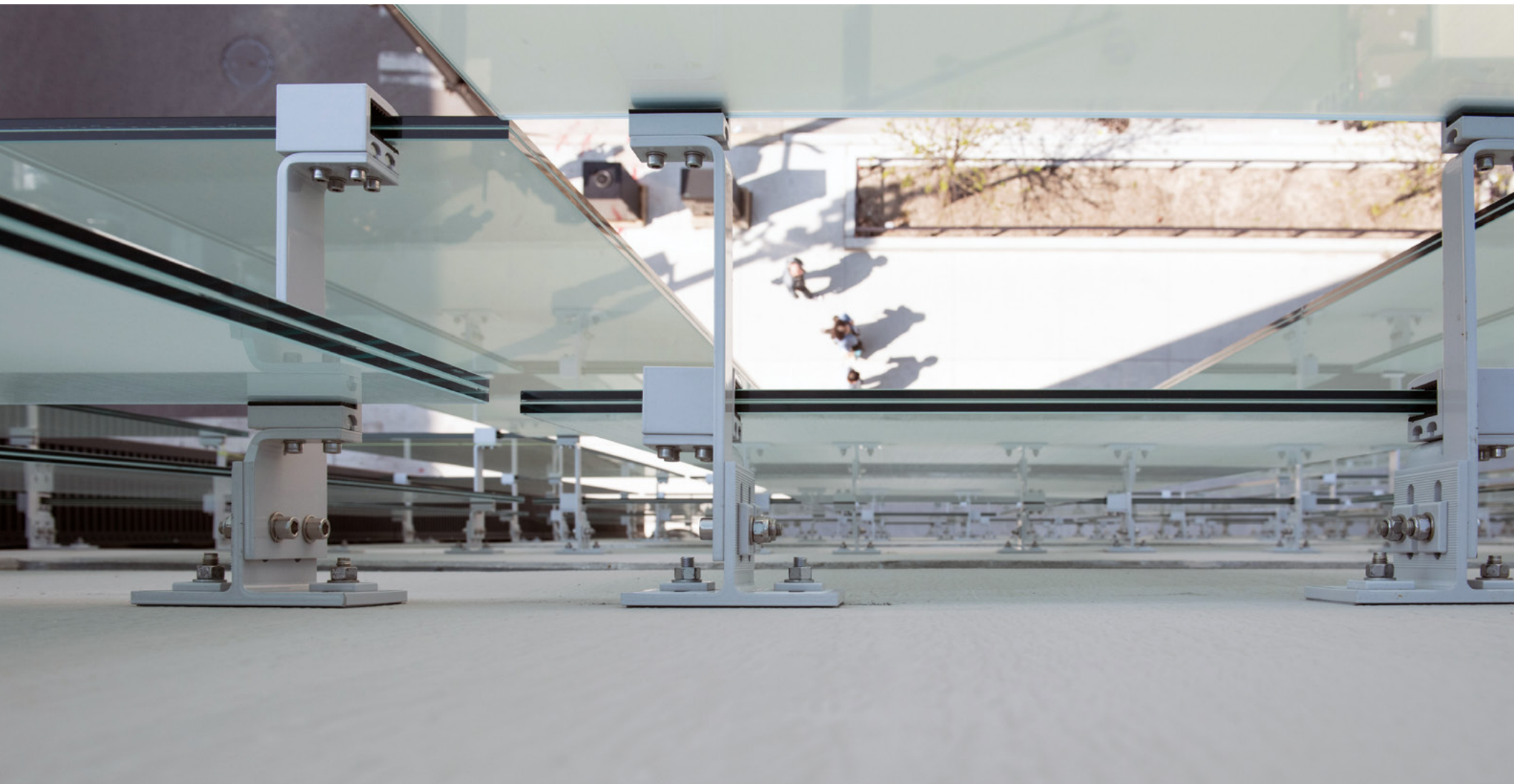
Detail top-down view of "staggered" north/south elevation.
