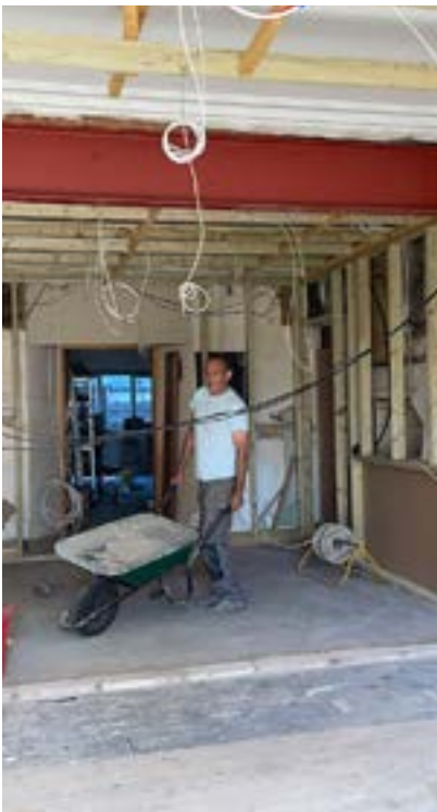
Installing the 4.5m RSJ
