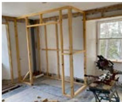
Building the new shower rooms
