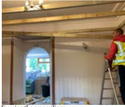
Framing the new ceilings
