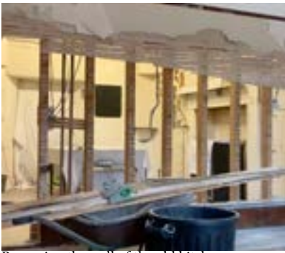
Removing the wall of the old kitchen
