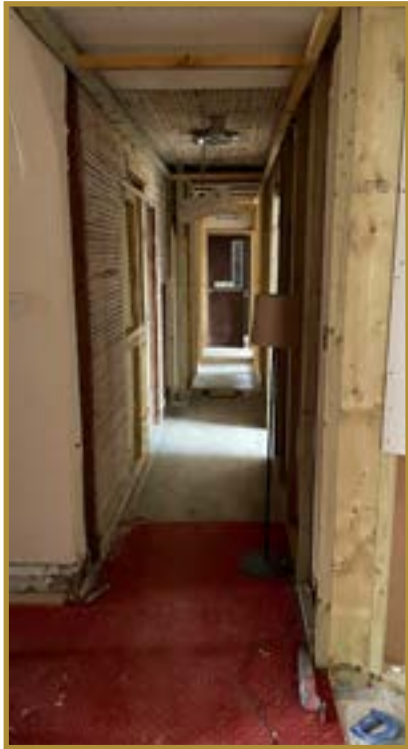
Lining the corridors
