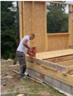
Building all the kits on site
