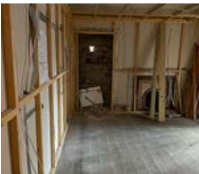
Lining all the inner walls
