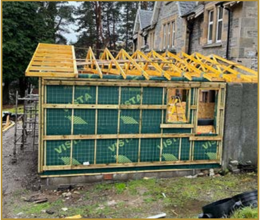
The extension with the trusses installed
