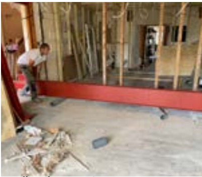
Installing the 4.5m RSJ
