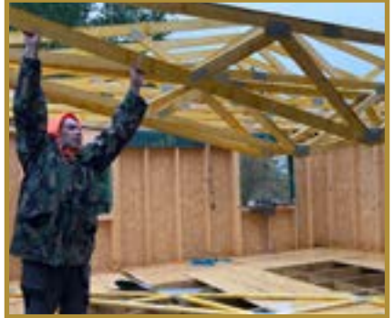
The trusses going up
