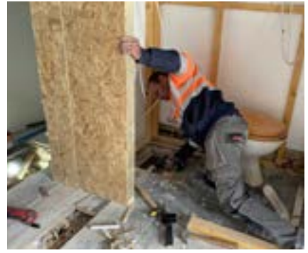
Fitting new water pipes
