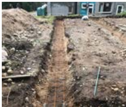
Preparing the foundations trench
