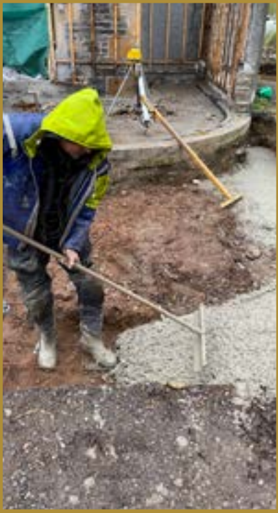
Nick laying the concrete for the extension
