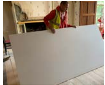
Over 100 sheets of plasterboard carried in
