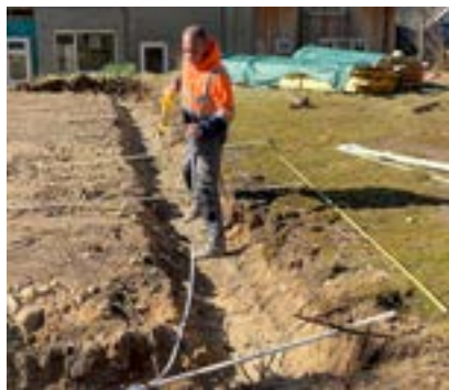
Measuring out the foundations
