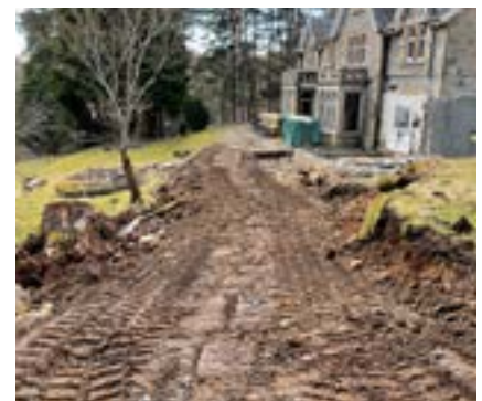
Creating the new drive way
