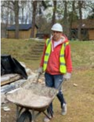
Many tons of materials were shifted
