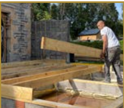
Building the floor for the extension
