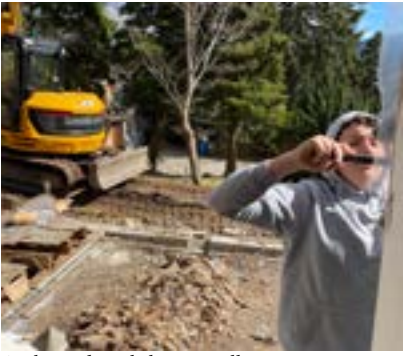
Anthony demolishing a wall
