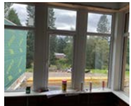
Over 50 new windows installed
