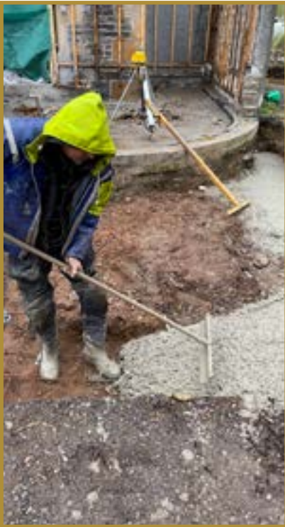
Nick laying the concrete for the extension
