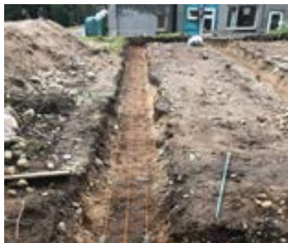
Preparing the foundations trench
