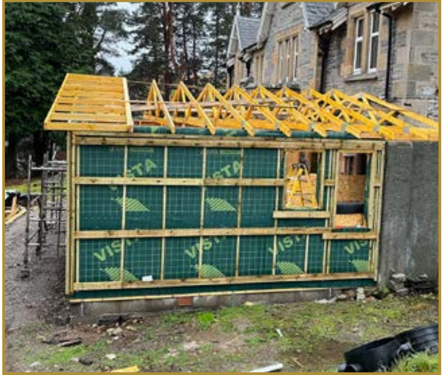
The extension with the trusses installed
