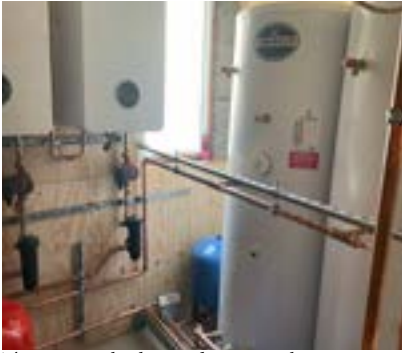
The new gas boilers and water tanks
