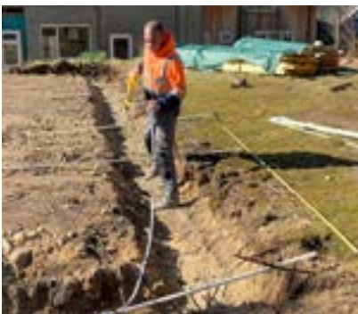
Measuring out the foundations
