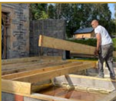
Building the floor for the extension
