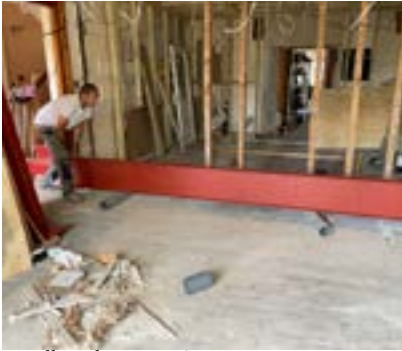
Installing the 4.5m RSJ
