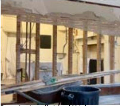
Removing the wall of the old kitchen
