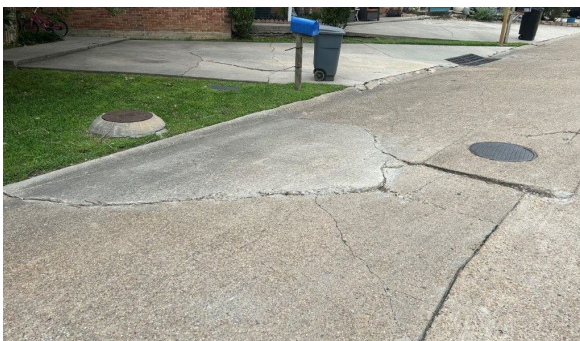
Area 3B with damage around storm manhole. Pavement has settled 2" which requires replacement.
