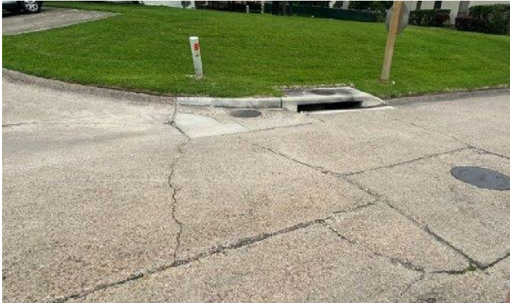
Area 1: Cracking around storm MH and inlet
