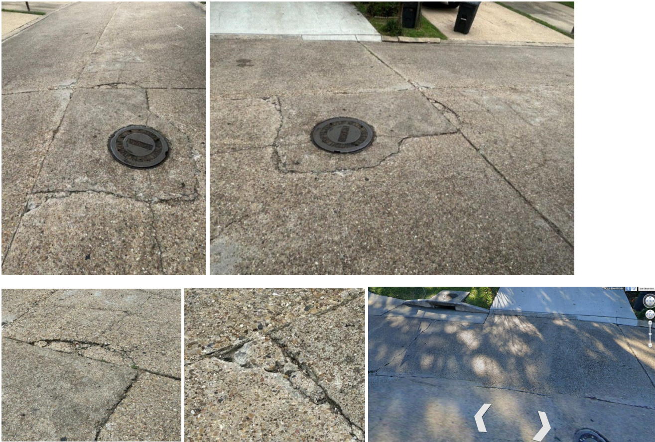
Area 21 on Knollcrest. Irregularly shaped manhole apron with concrete cracking and chipping around the perimeter.
