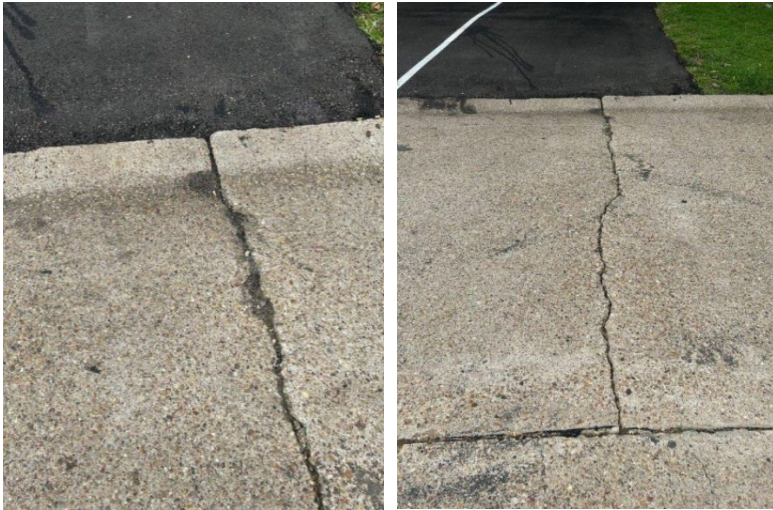
Area 19 on Glenview has a significant crack that will allow infiltration.
