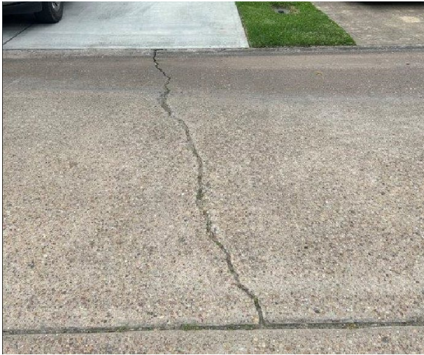
Area 4 has a 3/4" wide crack in concrete on Knollcrest Dr.
