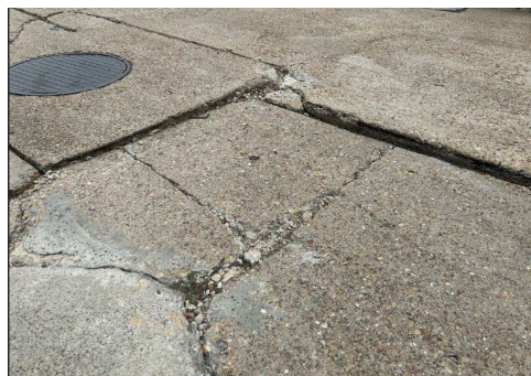
Area 3B with damage around storm manhole. Pavement has settled 2" which requires replacement.
