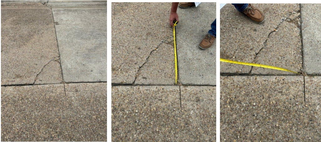
Area 17 with broken corners and a settled portion of a panel
