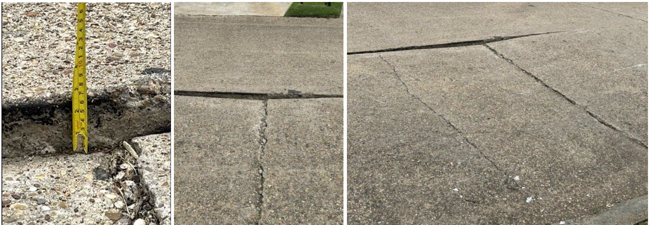
Area 18. Three-inch settled and cracked panel. The panel has 3 significant cracks in the pavement.
