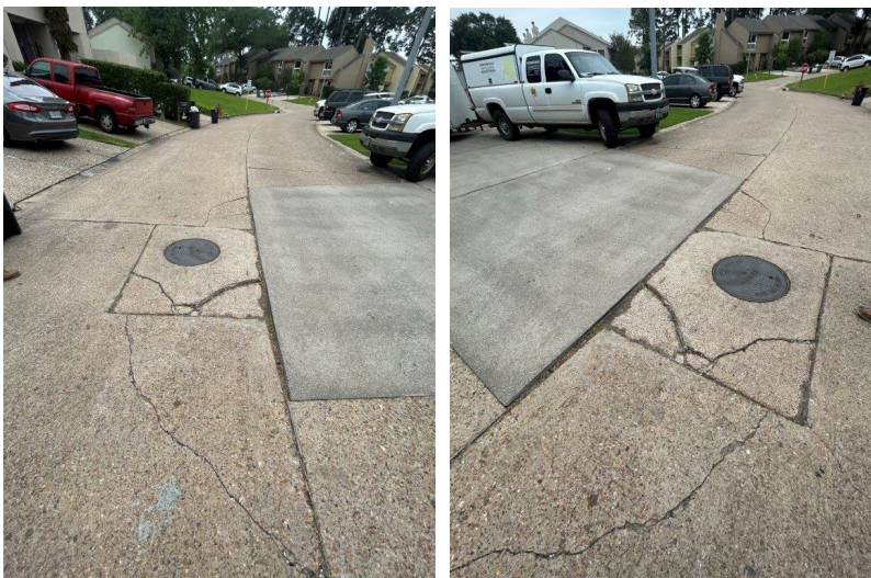
Area 11. Damage around storm MH.
