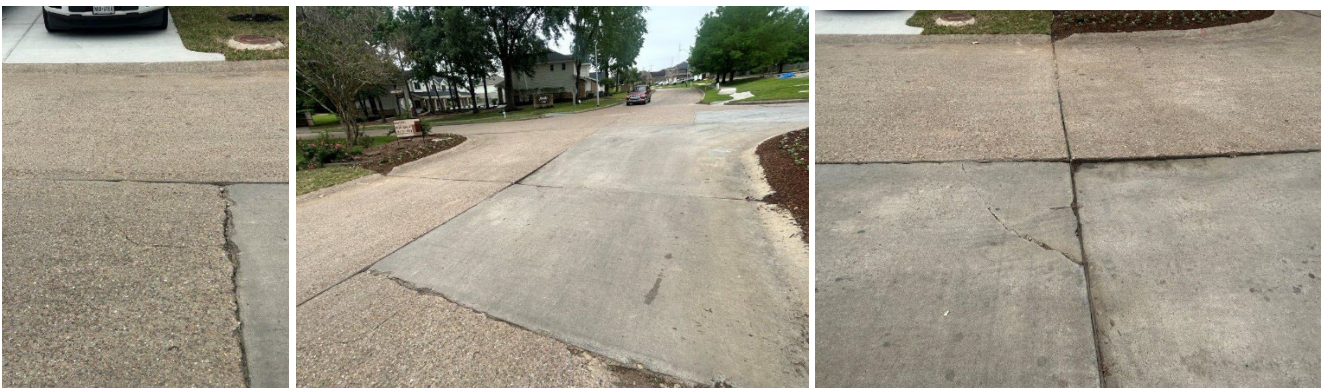
Area 16 with a jagged edge butt joint, 2" settled area, cracks, and broken corners.
