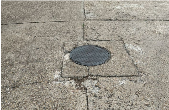
Area 3A with broken Apron around MH
