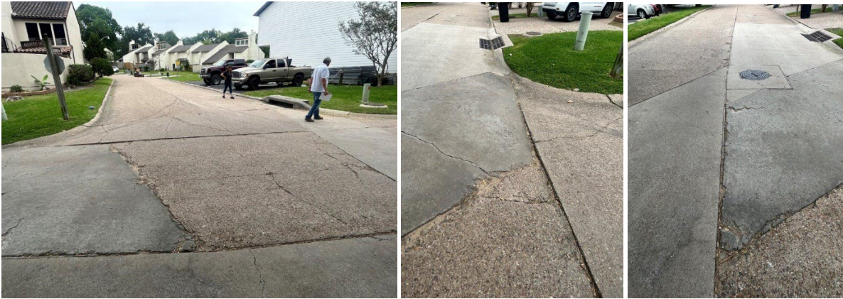
Area 14. Concrete is cracked, broken, and settling at the intersection.
