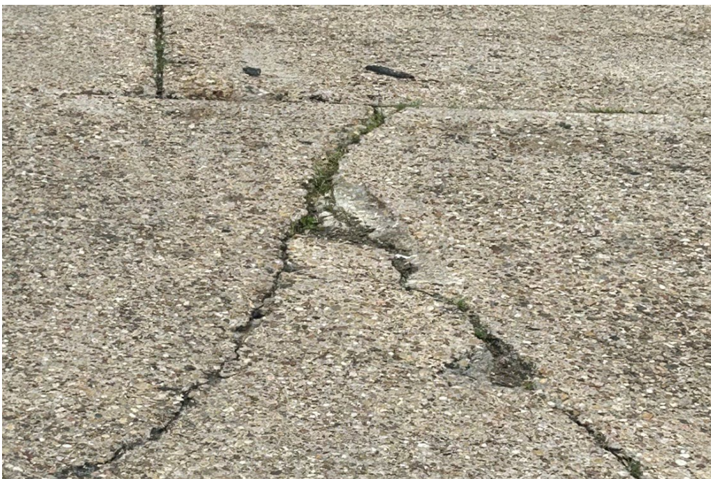
Area 22 on Knollcrest has merging cracks leading to chipping away from frequent vehicular loads and impact from tires.
