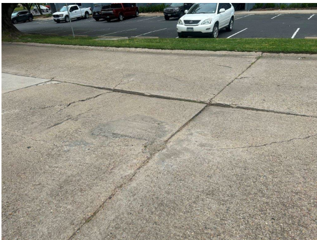
Area 13 on Lakewood Drive has settled 2" at the centerline of the street.
