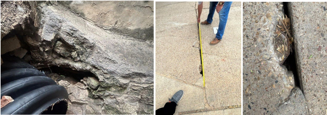
Area 14. A failed seal around the storm pipe has led to voids under the paving and chipping off material at the edges.
