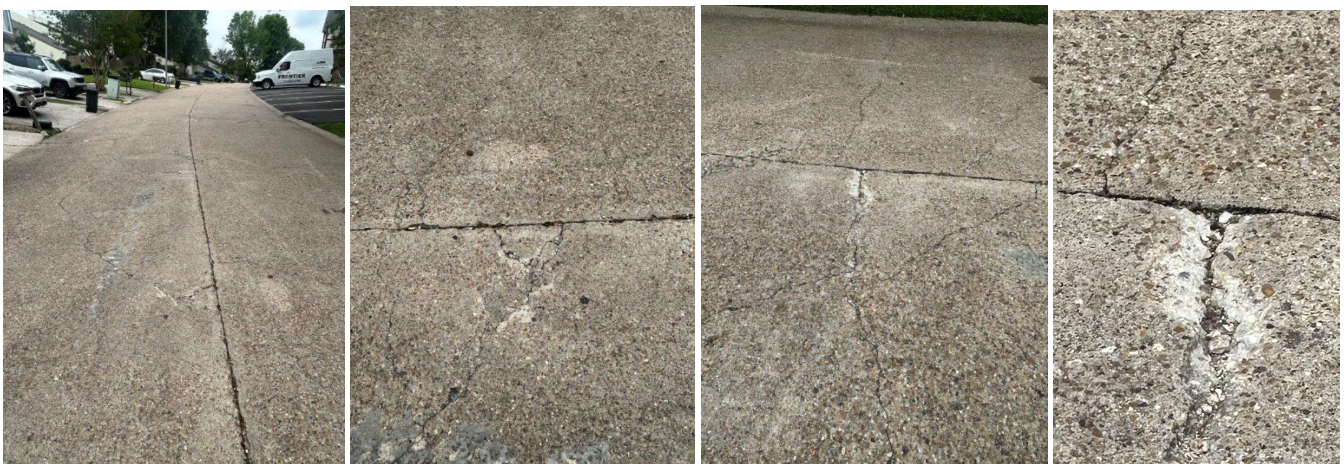
Area 20 on Glenview near Knollcrest has a significant area of cracking which has led to surface damage.
