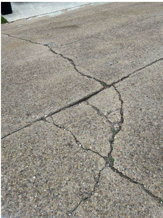
Area 2 broken concrete with 1" settled pavement.
