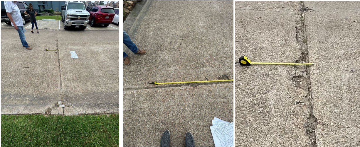
Area 10. Damage at the edge of the joint needs repair to prevent more damage.
