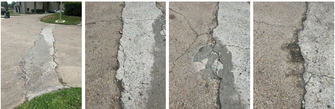
Area 5. Concrete chipped out and replaced without saw cutting at northern end of Knollcrest.
