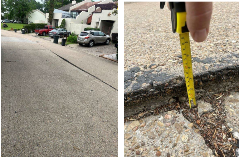
Area 12 on Lakewood Drive has settled 3" as measured relative to the adjacent panel.
