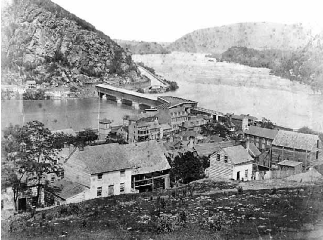
B&O Bridge, Ferry Lot / Point, and Lower Town (1859) (Viewed from Upper Town)
