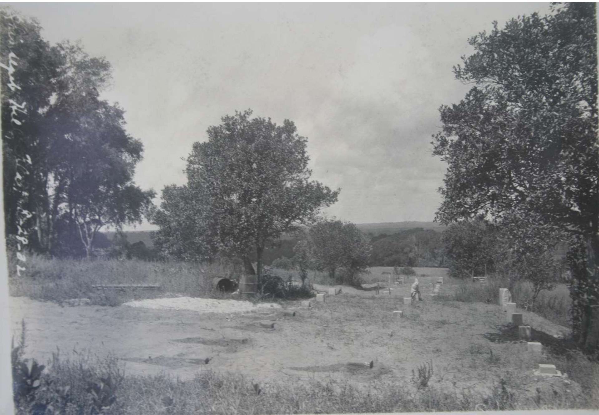
Foundation for Hen Laying House, August 28, 1932
