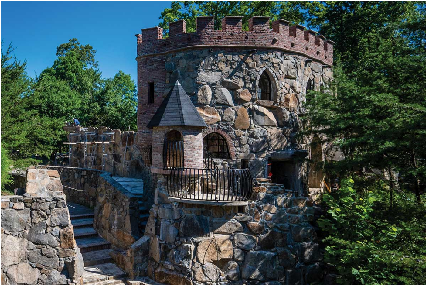
The castle the Knops are building is made of local stone, reclaimed highway construction material, parts of old buildings, utility poles, and other reused things. (Photo by Will Schermerhorn)
