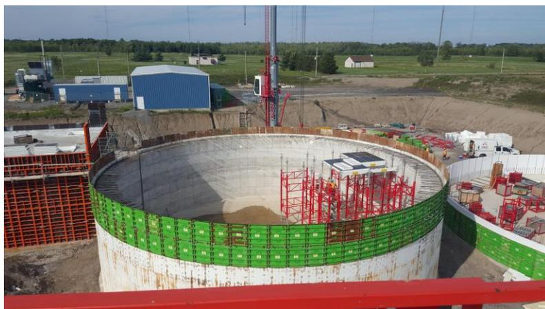
facility received TSSA approval in mid-July. On the 20<sup>th</sup> of July, the tanks were loaded with 300,000 gallons of manure to start the process, and the facility began producing and flaring low-quality biogas about 10 days later. On August 10<sup>th</sup>, they officially started producing electricity and generating revenue.
