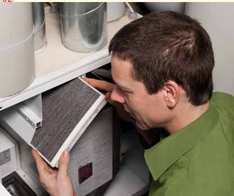
Replacing the filter of a ventilation unit.
