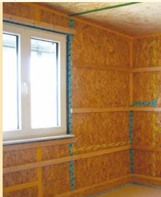
Airtight connections between wood composite boards
