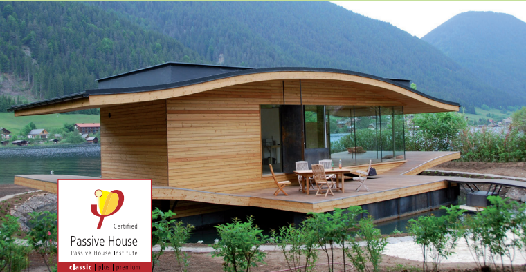
Single family home in Italy | Michael Tribus Architecture | Photo © Michael Tribus
