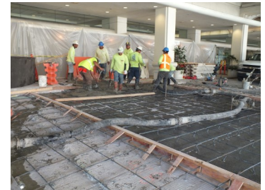
Forming and placement of concrete to adjust grades
