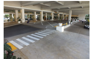
Completed grade adjustments that meet ADAAG regs.
