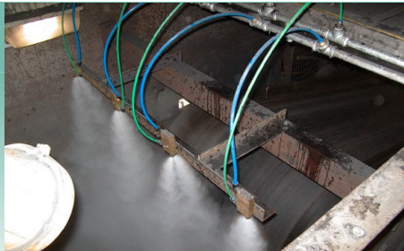
Typical Sonic Dust Suppression Installation At Conveyor Discharge
