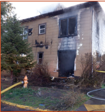
Cause of this building fire in the top right unit was deemed “undetermined”.
