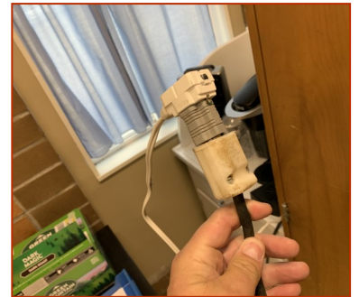
Two extension cords connected by an electrical adapter. Extension cords are for TEMPORARY use only, not a substitute for permanent wiring.
