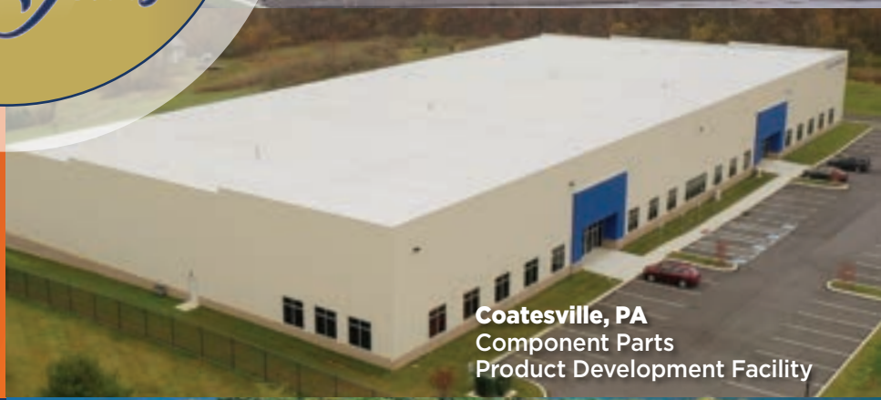
Coatesville, PA Lifts Product Development Facility
