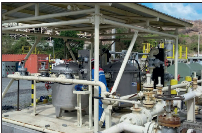
Changing 1 \mu m high flow filter elements HF900 after 16.000.000 l.
