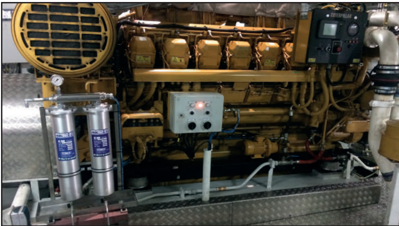
AL600 double system for oil on a generator
