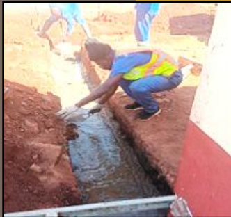
Description of Picture: Construction taking place at Thyolo Prison
