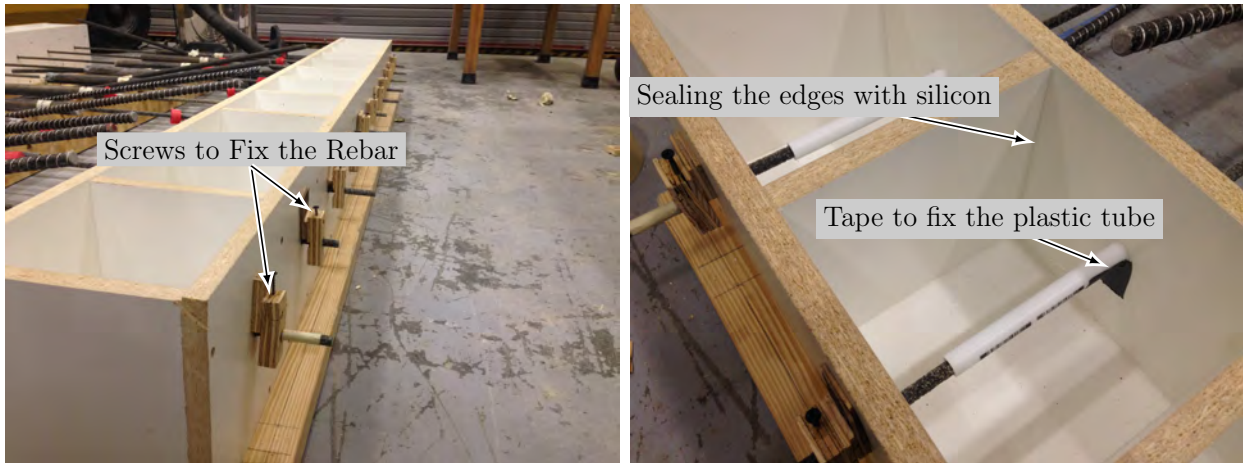
Figure 4.18: Fixing the rebar and the plastic tube
