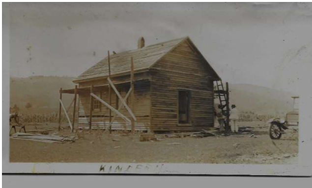
Kinderhook School Under Construction
