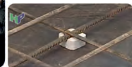
Application of Slab Cover Block
