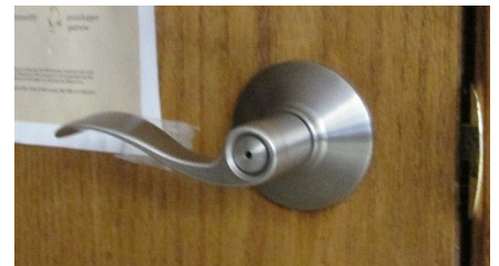
Replaced doorknobs with lever handles
