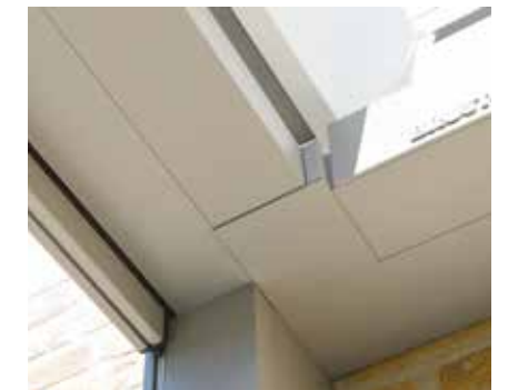
Waterafvoer via goot direct in steunpaal
