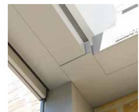
Waterafvoer via goot direct in steunpaal
