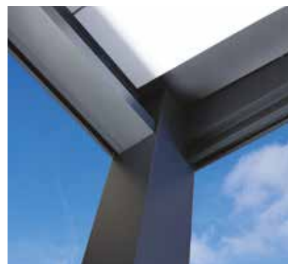
Waterafvoer via goot direct in steunpaal
