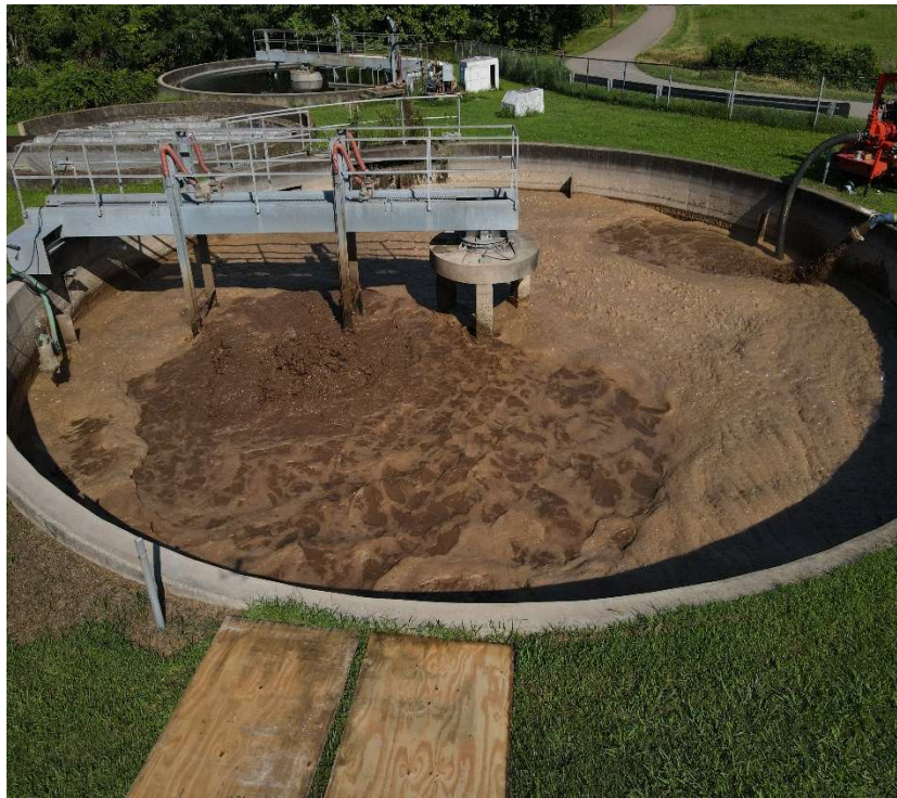
Figure 1 Picture taken during the premixing stage in the startup of G3 Wastewater Tech Process
