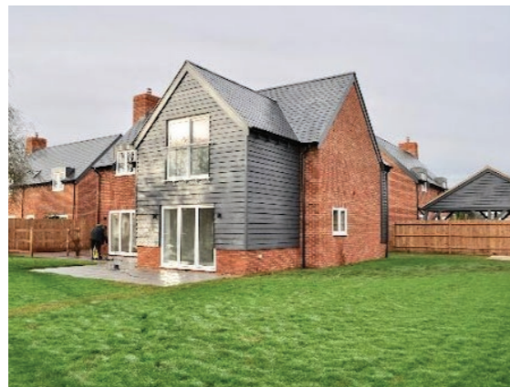
Manor View, Steeple Claydon Completed January 2022
