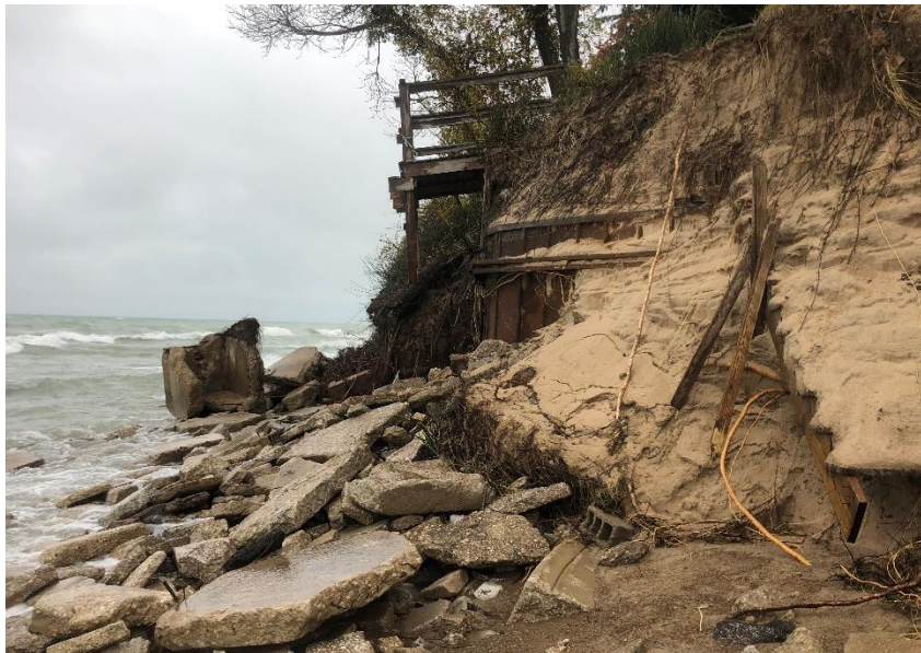
Figure 4: Photo of Stop 43 Seawall Facing North, 10/29/19
