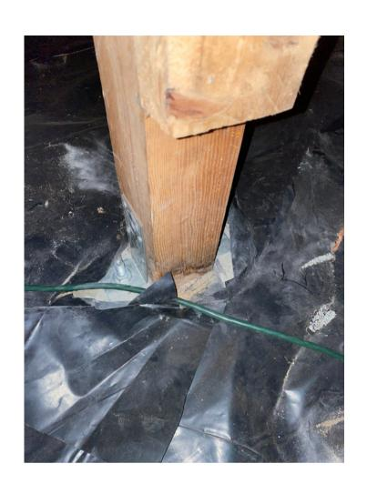
3 posts secured by contractor. No sag or compromise to floor joists was noted.
