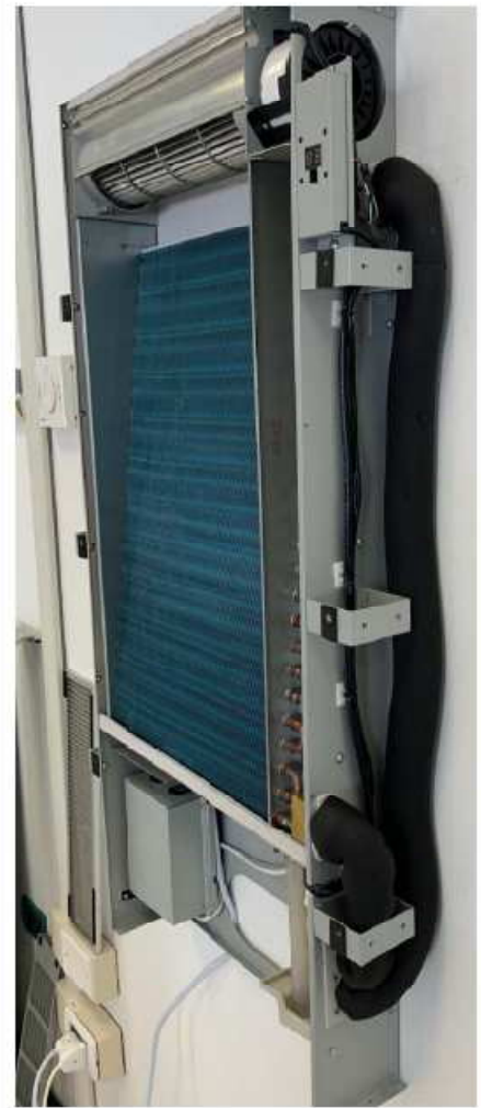
PUT INSULATION IN ALL THE EXTERNAL PIPE
