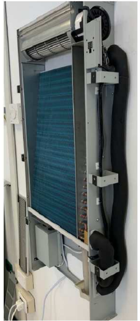
PUT INSULATION IN ALL THE EXTERNAL PIPE
