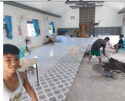
Work delayed by typhoon, but now good progress
