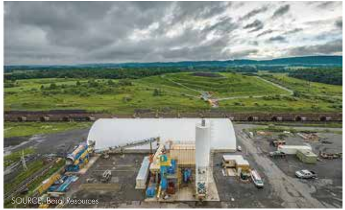
Santee Cooper's Winyah Generation Station (I) uses the SEFA Group's Staged Turbulent Air Reactor (STAR) technology to reclaim coal ash from on-site ponds for its primary raw feed. Dry stack harvesting is carried out (r) at Boral Resources' Washingtonville, Pennsylvania, monofill.
