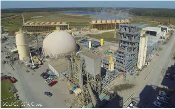
Santee Cooper's Winyah Generation Station (I) uses the SEFA Group's Staged Turbulent Air Reactor (STAR) technology to reclaim coal ash from on-site ponds for its primary raw feed. Dry stack harvesting is carried out (r) at Boral Resources' Washingtonville, Pennsylvania, monofill.
