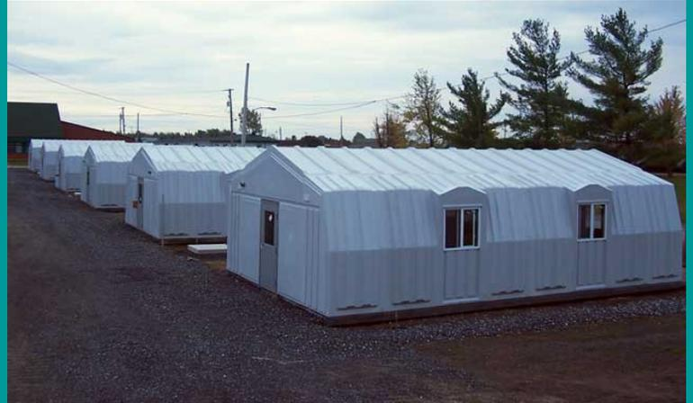
A resounding success, these buildings hold up to all the elements inside and out. The buildings are portable if required for relocating at a later time. RM Products fiberglass modular enclosures allow for expansion, by simply adding side-wall panels the buildings size can increase in four foot increments, as required.
