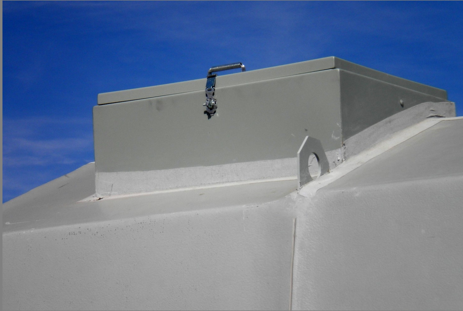
Roof Hatch & Lifting Eye
