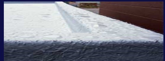
Fiberglass pan (above) holds spilled liquid, it is mounted to modular building and then sealed with fiberglass for seamless flow from floor to ceiling.
