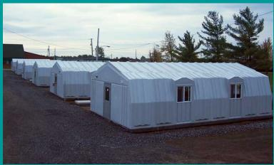
A resounding success, these buildings hold up to all the elements inside and out. The buildings are portable if required for relocating at a later time. RM Products fiberglass modular enclosures allow for expansion, by simply adding side-wall panels the buildings size can increase in four foot increments, as required.
