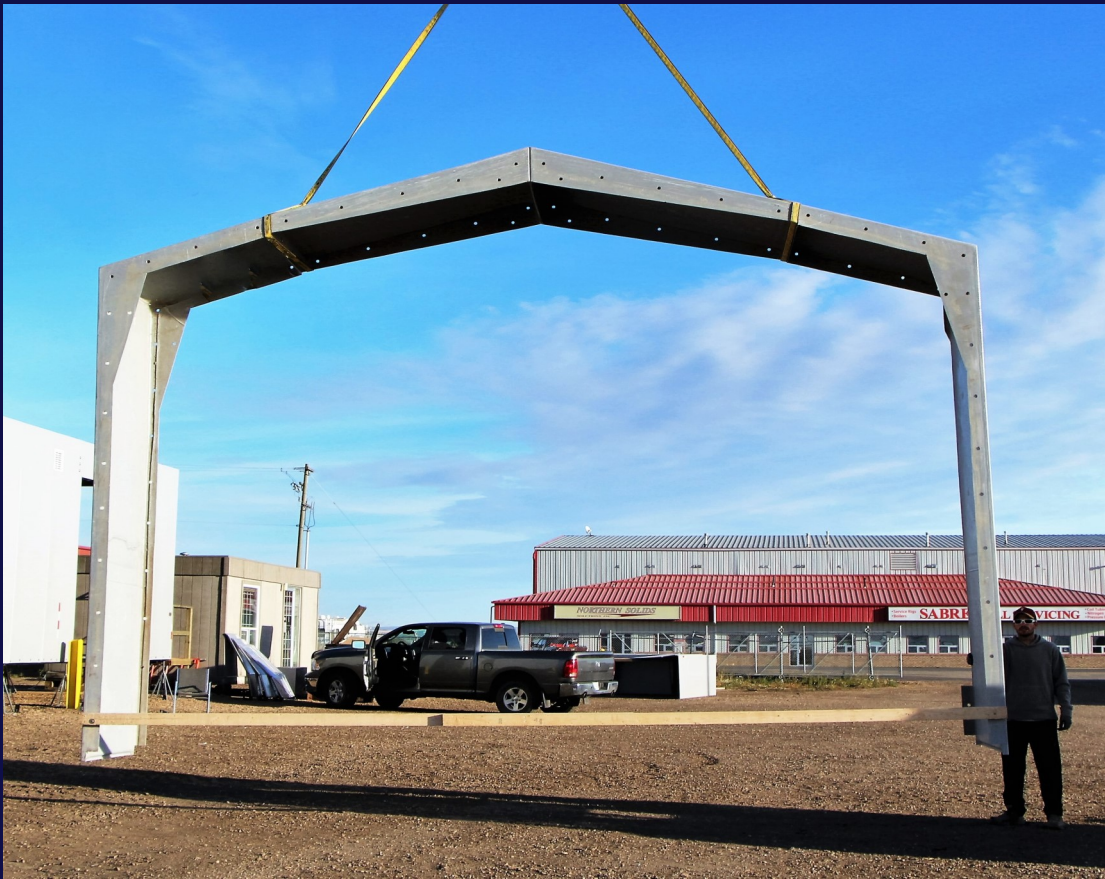
Sections are easily lifted by an extendable forklift or crane.
