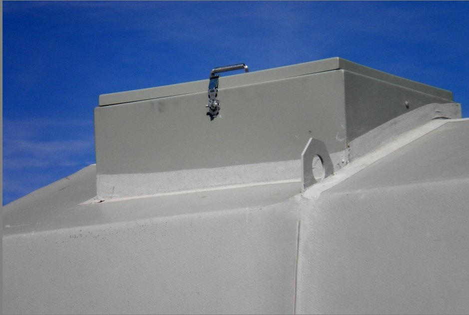
Roof Hatch & Lifting Eye
