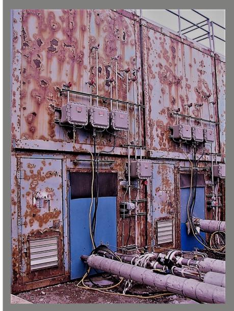
No longer have to look like this over time. Corrosion from the Arctic Ocean destroys steel wellhouses, creates an unsafe building and an environmental problem.
