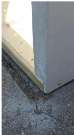
Step 5: When the panel is snug to the end of the base drill and bolt to the base/floor using lag bolts supplied at approximately 16" O.C.
