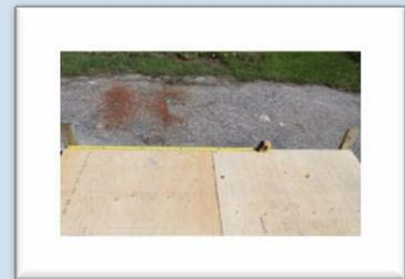
**NOTE: The "LEVEL" base is critical for proper door operation.**
