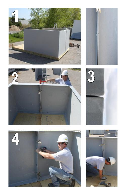
Step 1: Layout rear section next to base (a section is two side wall panels together to make a U shape). Be sure to have the drilled holes of the roof section facing down. There will be no holes in the side facing up.
