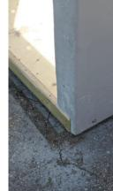
Step 5: When the panel is snug to the end of the base drill and bolt to the base/floor using lag bolts supplied at approximately 16" O.C.
