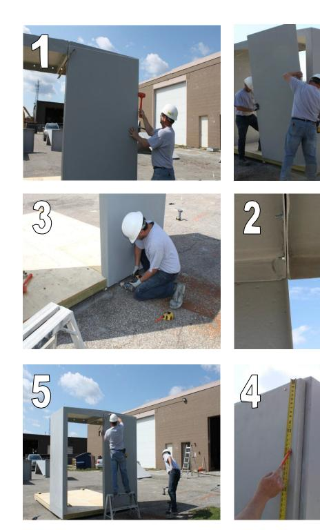
Step 1: Set one of the rear panels in place and clamp along the internal flange, in the top corner of the rear panel.
