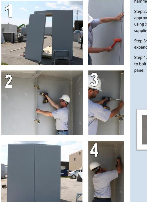
Step 1: Set other rear panel in place, align using a dead blow hammer and clamp.
