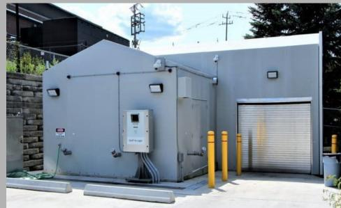
All man doors are fiberglass, the roll up door has non-corrosive features. All hardware is stainless.
