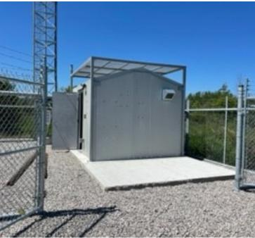
RM's ice rakes are custom made for our modular buildings. The ice rakes break the ice up if it falls from the roof of the building.
