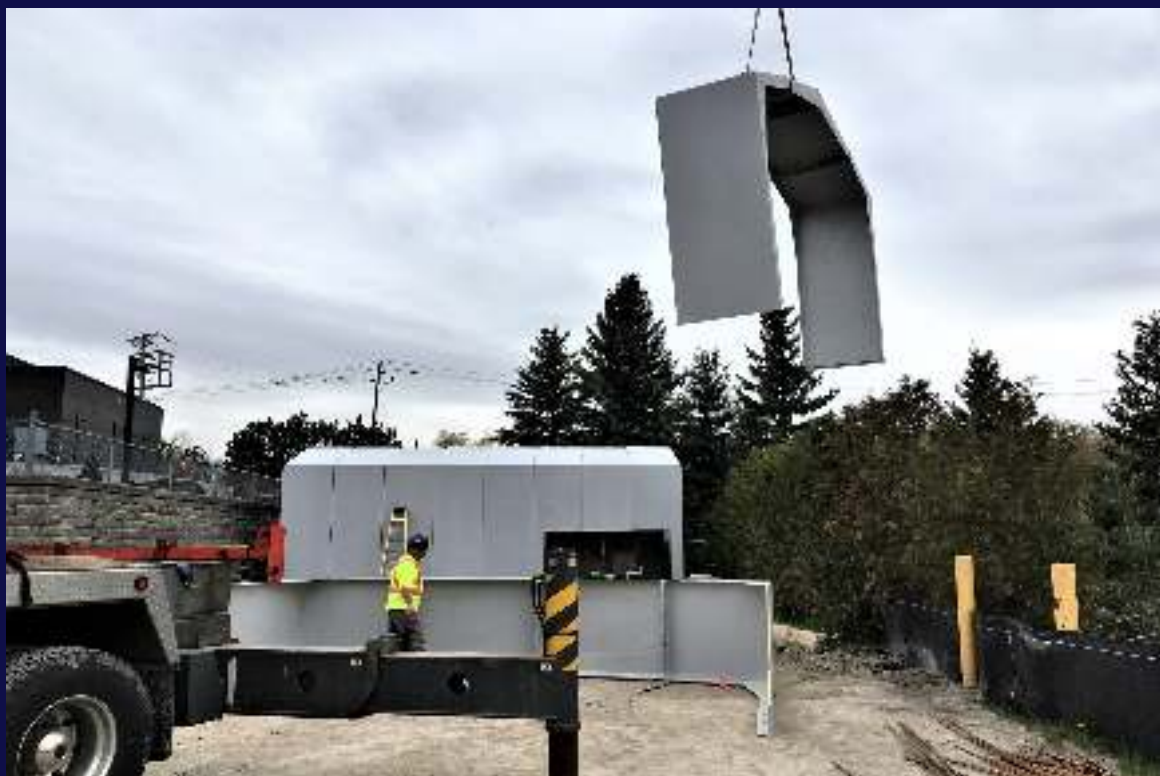
Sections are easily lifted by an extendable forklift or crane.
